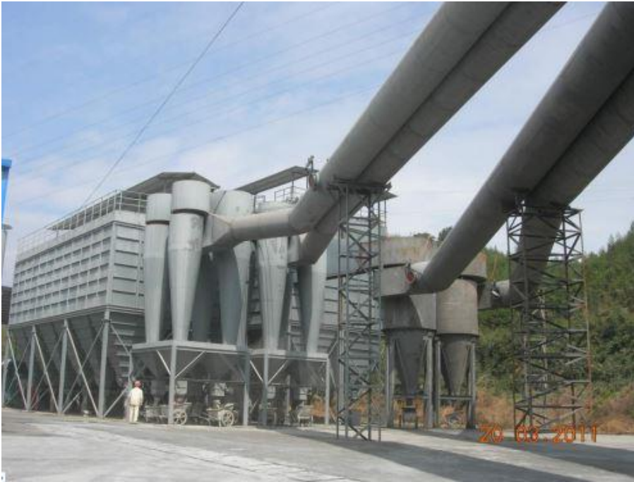
In 2009, the high carbon ferrochrome dust removal equipment on the scene
